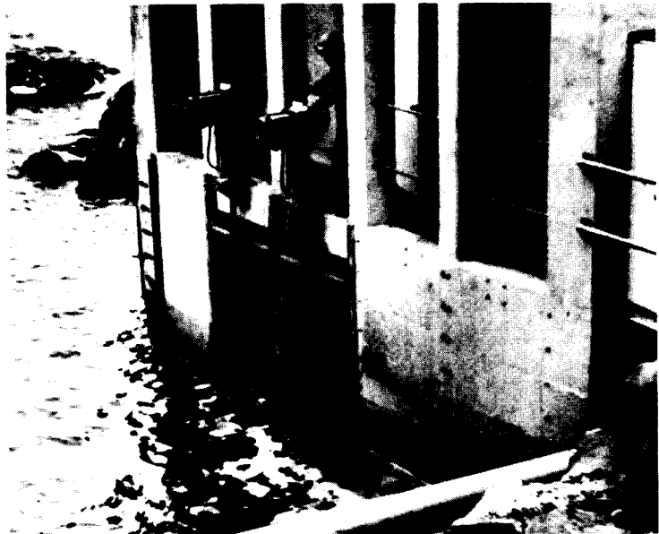
Photo showing offset electric operated slide gate lifts at the inlet of a pump station for sea water.
