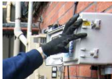
IP66/NEMA 4X panel offers protection against entry of dust or water during meter programming
